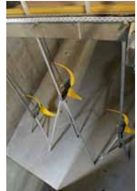
The guide bar system makes mixers easily accessible.
